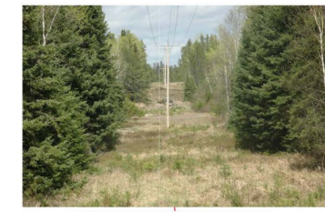
HYDRO DISTRIBUTION CORRIDOR
