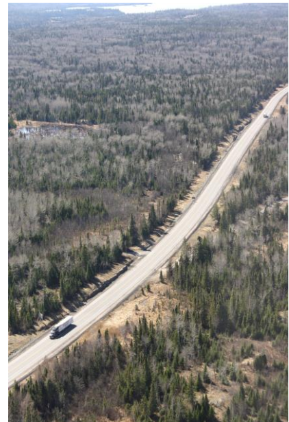
Study Area between Gundy Lake Road and Baubee Lake
